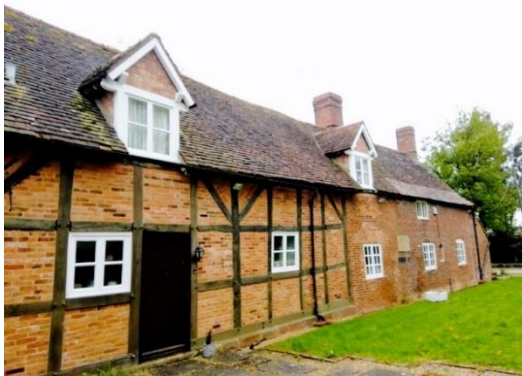
Moat House Cottage in Canley, birthplace of Sir Henry, today a private residence Photo: John Marshall
