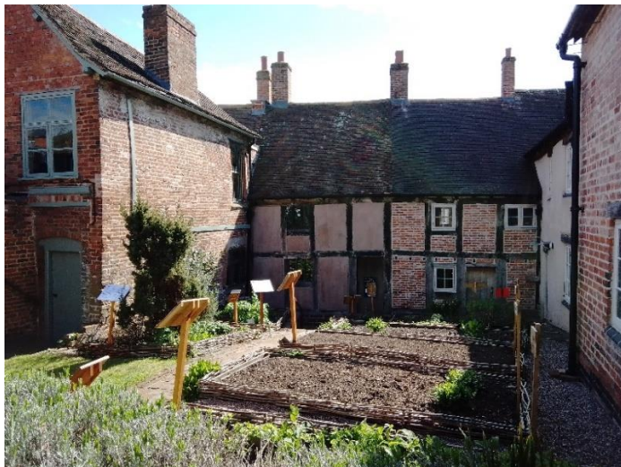
Rear of the Weaver's House, with its medieval garden
