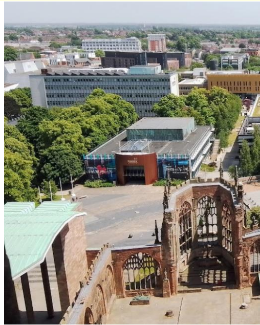
As it was: the Alan Berry Building once occupied a prime location in front of the Cathedral.
