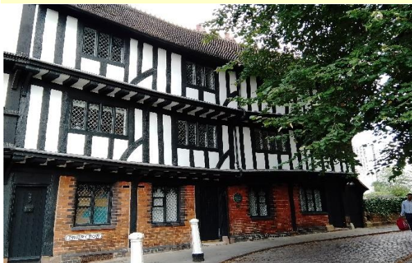
Lychgate Cottages, Priory Row, one of the properties restored by Historic Coventry Trust
