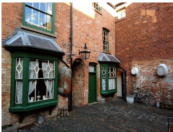
Some of the inner houses in Court 15, Birmingham. The bay windows indicate a higher class of design than many similar properties, but the rooms were still tiny and walls were only one brick thick. Photos: John Marshall
