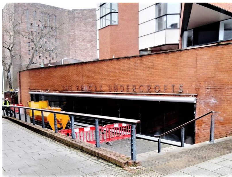
Work underway at the Priory Undercrofts this month
