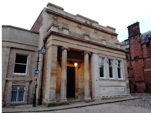
Drapers Hall – now wonderfully restored after standing empty for 30 years.
