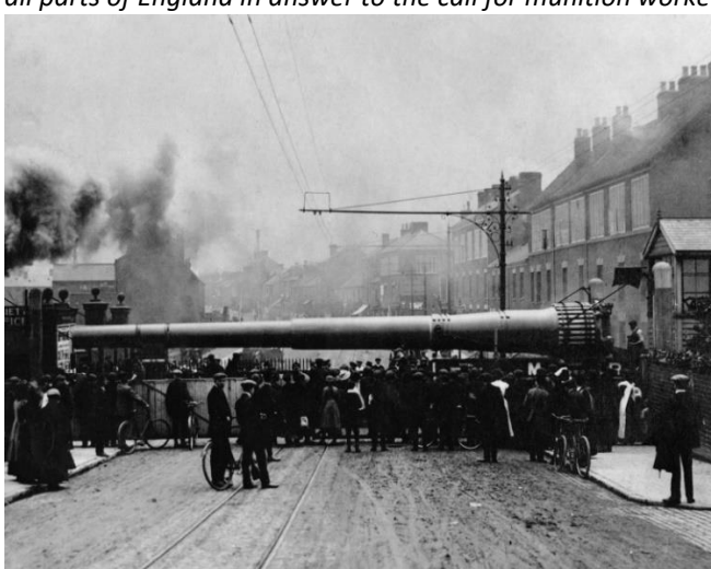
A giant naval gun barrel is taken by rail across Stoney Stanton Road from the Ordnance Works factory on the right, 1912
