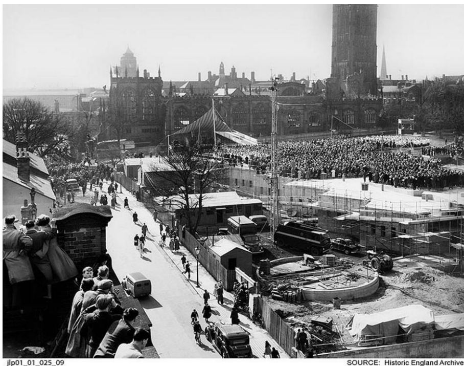
Crowds gather to watch the foundation stone laying ceremony in March 1956
