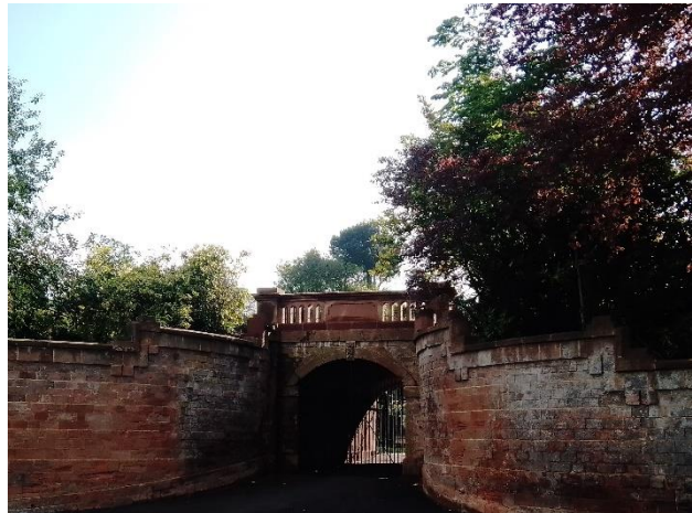
Revealed at last: the old gated entrance tunnel is now visible again from London Road
