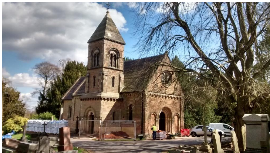
Work in progress this month at the Norman-style Anglican Chapel
