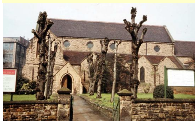
All Saints Church, pictured in c1970, shortly before its demolition. Note the distinctive round windows providing light to the clerestory level of the nave, and the gabled south aisle. The pollarded trees are still there today, now much larger and in full leaf. Photo: City Council conservation area team
