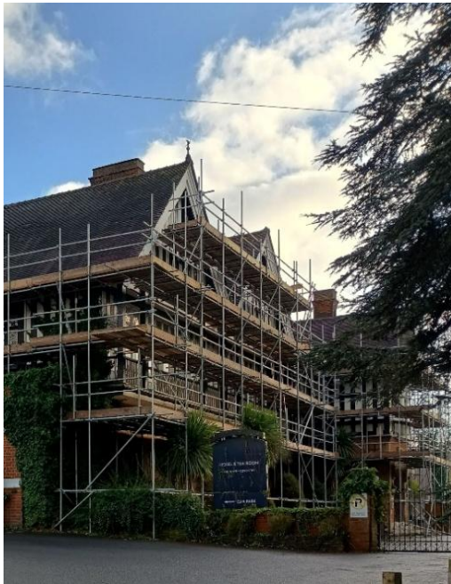
Exciting signs of progress: restoration begins Photo: John Marshall
