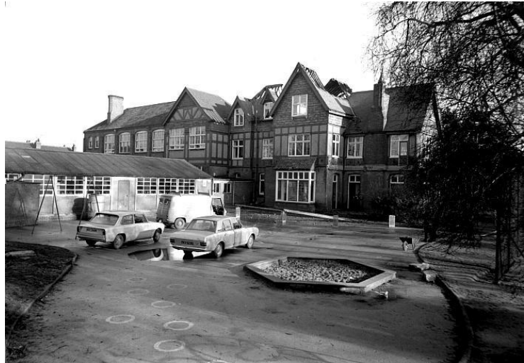
A rear view of the building immediately after the fire in 1972, showing damage to the roof and upper floors. The wing on the far left is an extension to the original house, probably added in 1926. After the fire, the wing on the right was demolished and the roof realigned. Photo courtesy of Rob Orland / Historic Coventry
