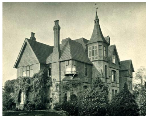
This view shows the original tower at the front and the south wing on the left.
