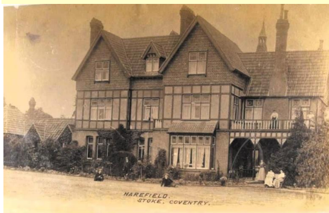
A rear view of Harefield House, the former Hope's Harbour, with its extensive garden lawns. It acquired its new name after 1895 and was destined to become the new Stoke Park School.
